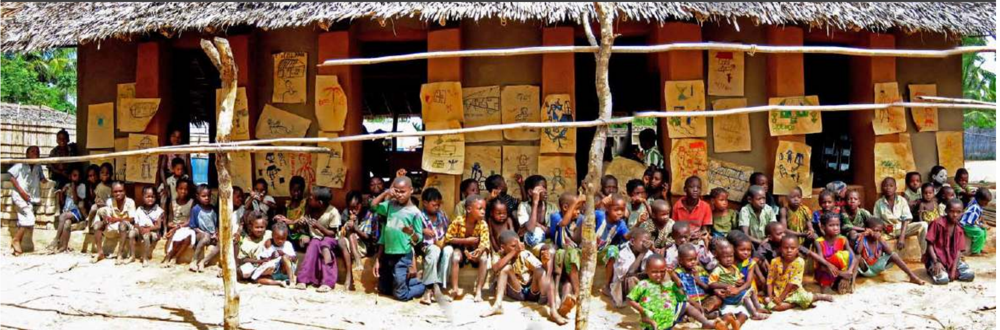
Completed ecologically-constructed community learning centre
