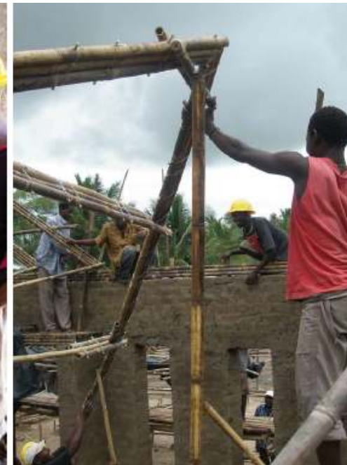
Youth apprentices learning how to develop improved bamboo framing systems, which utilise natural materials, such as cashew oil, to prevent pest attacks, and are formed into beams for additional strength
