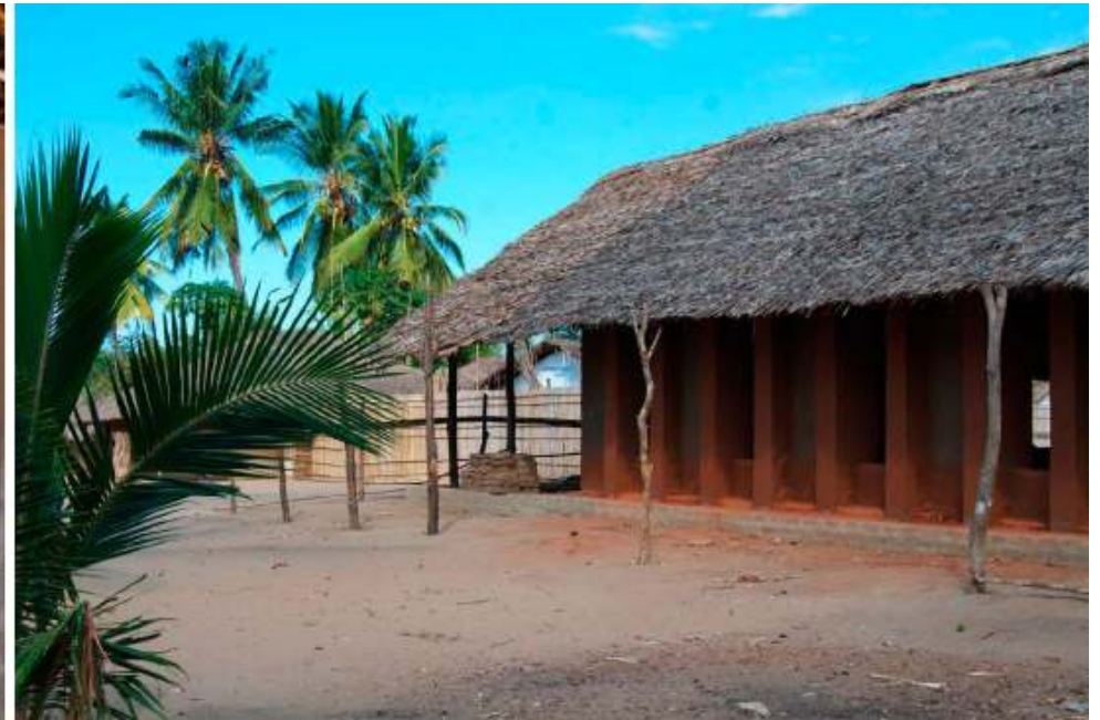
The structures feature foundations, thick mud blocks walls, and large roofing spans to accommodate bigger floor plans, all constructed sustainably with locally available materials
