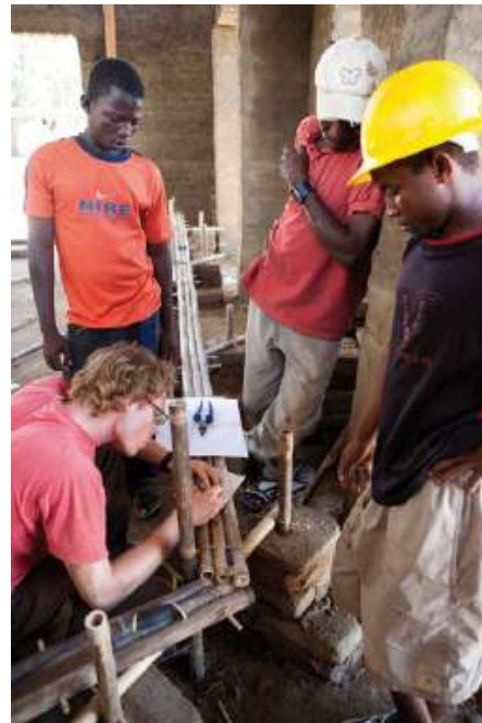
Youth apprentices learning how to develop improved bamboo framing systems, which utilise natural materials, such as cashew oil, to prevent pest attacks, and are formed into beams for additional strength
